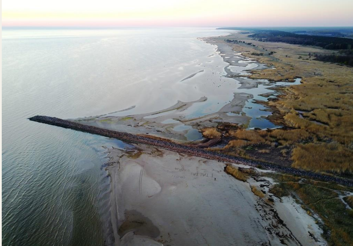
Fig. 2. Breakwater near Ainaži (Latvia)
